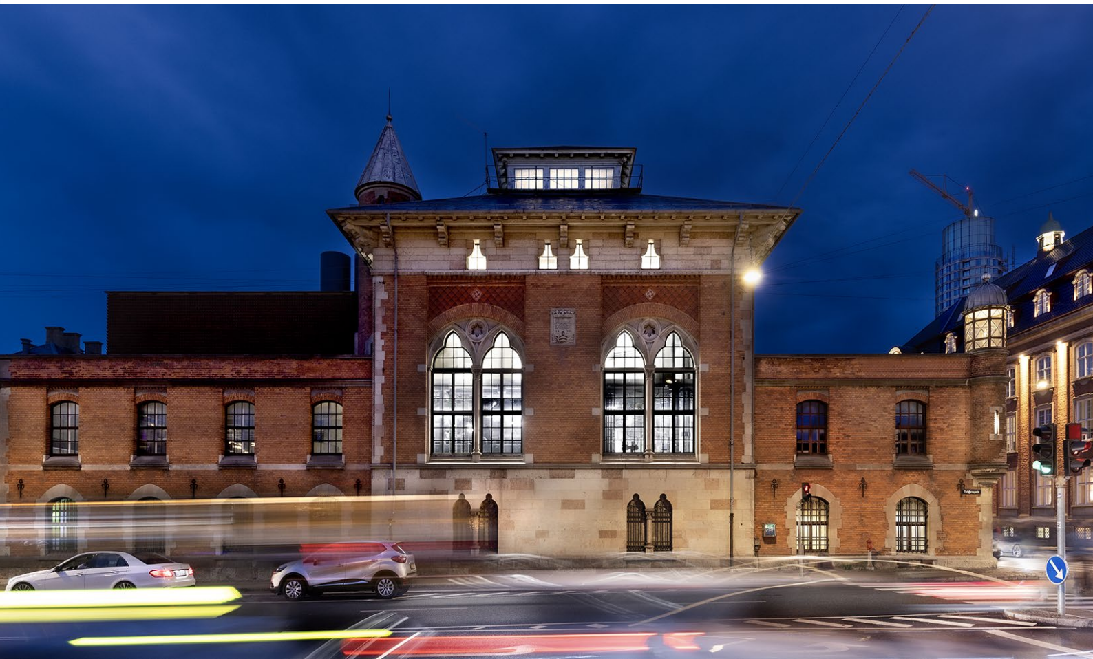
The three Fenagy CO 2 heat pumps are housed in a 126-year-old former power station in downtown Copenhagen. Photo credit: HOFOR and Fenagy
